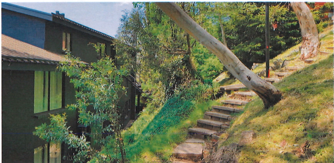
Figure 17: Rear of the existing building
