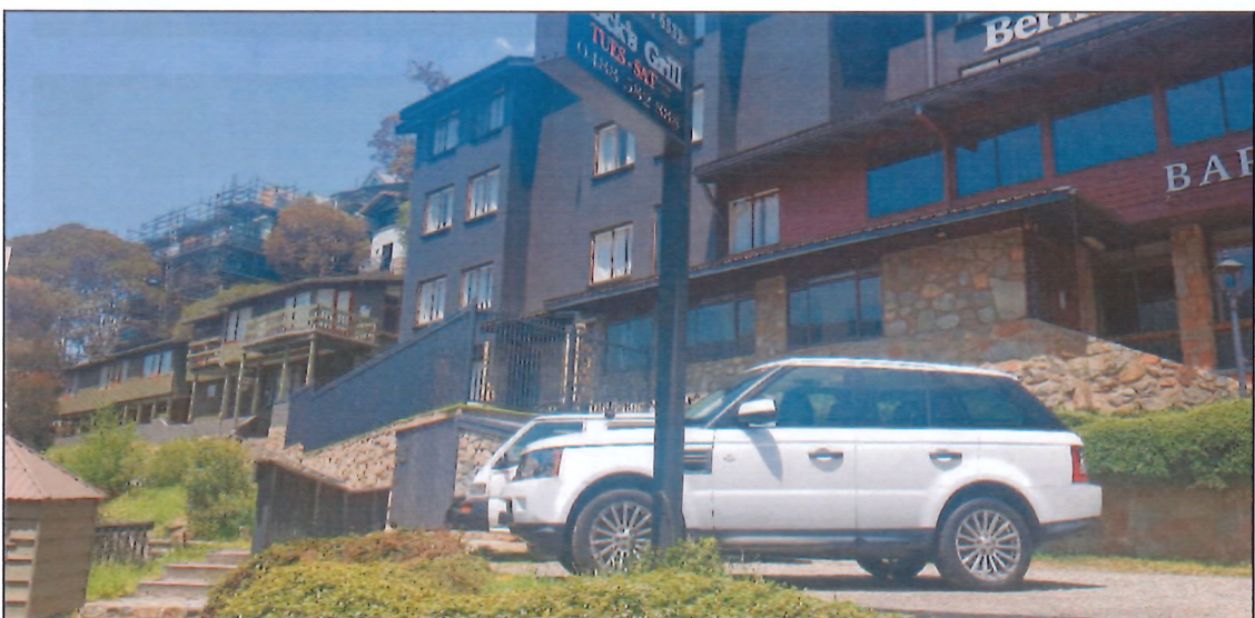
Figure 15:Image of adjoining development
