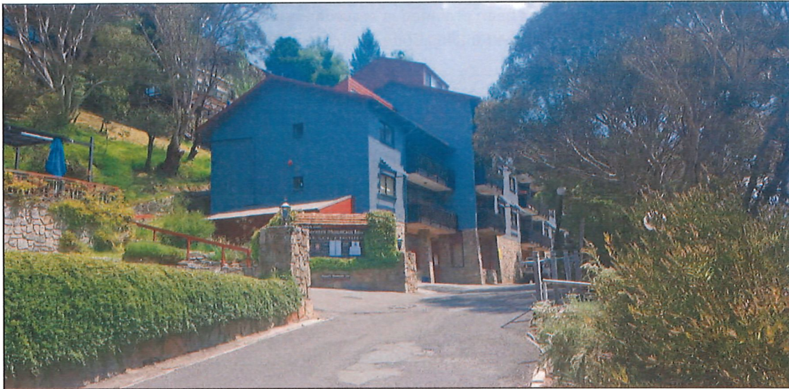
Figure 26: Image of existing access off Mowamba Place
