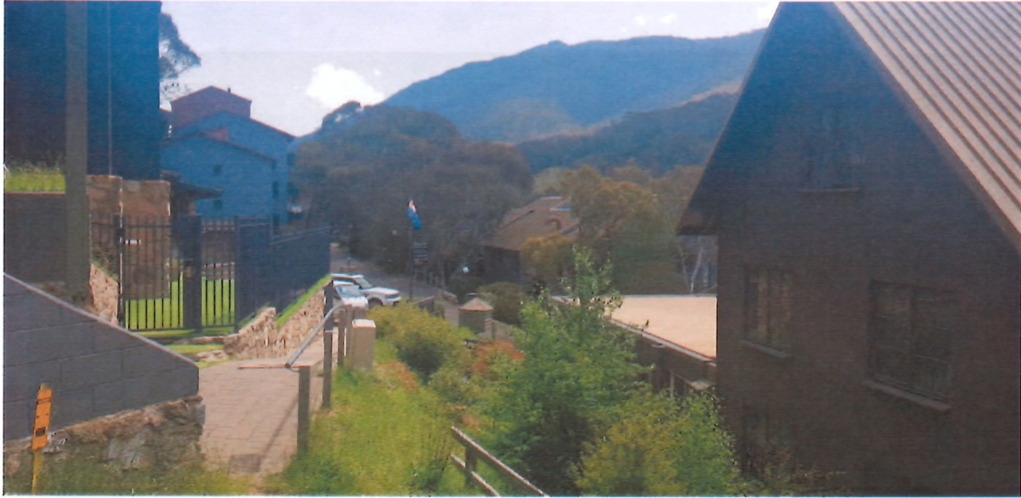
Figure 13:View from corner of exiting building looking west down Mowamba Place
